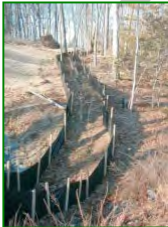
Typical Silt Fencing
