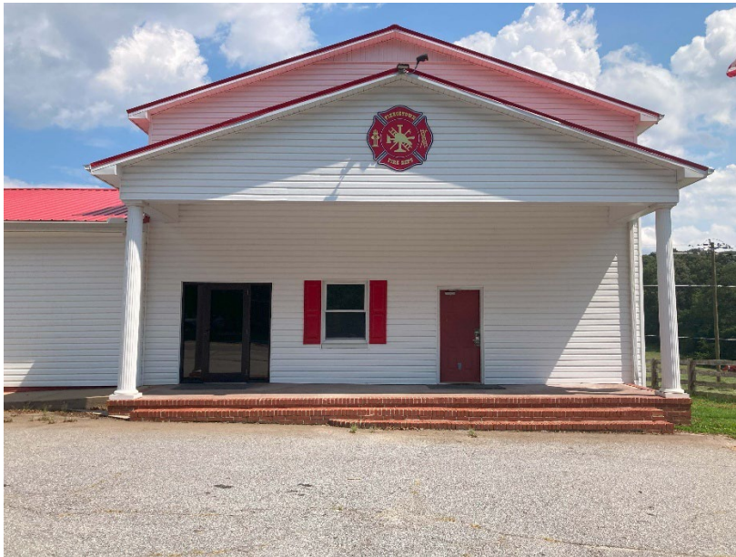
Piercetown Fire Station
