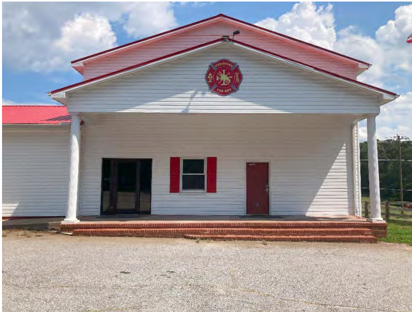
Piercetown Fire Station
