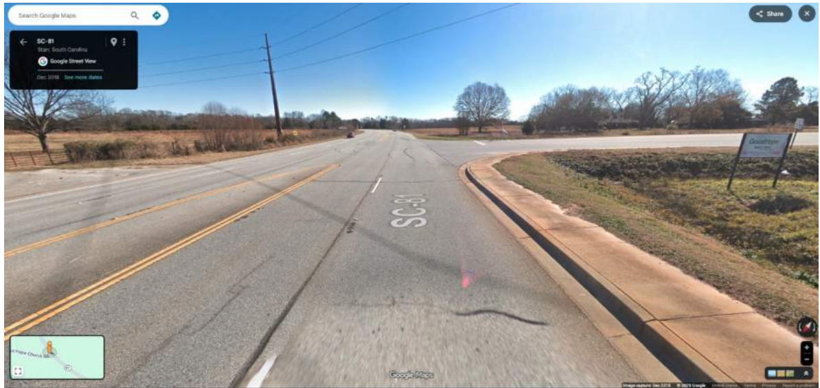
SC 81 at S-105 looking southeast
