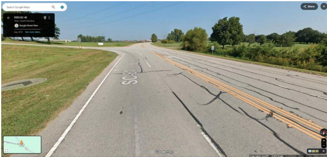
SC 81 at S-105 looking northwest
