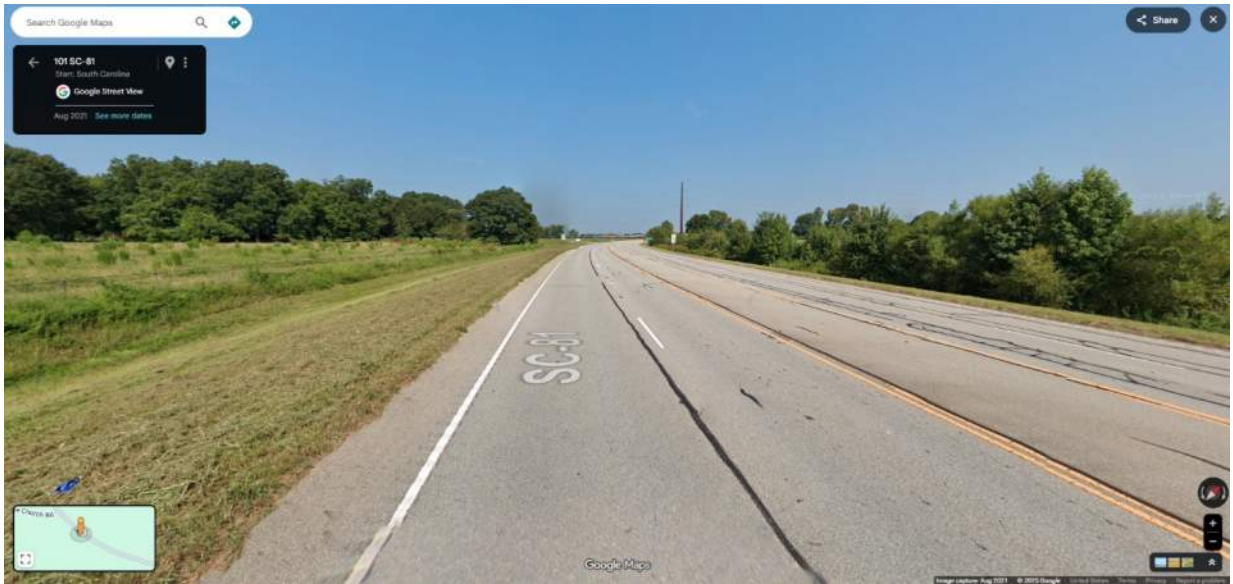
SC 81 at Car DW looking northwest
