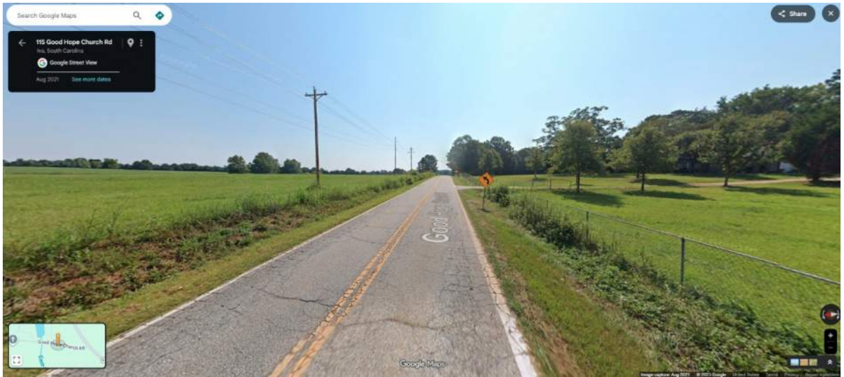
S-105 at Bus Driveway looking east
